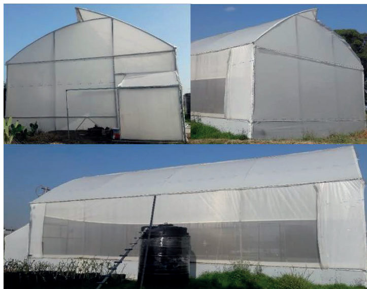
Figure 4. Sawtooth-type experimental greenhouse with drip irrigation located at Chapingo Autonomous University, 2016.
