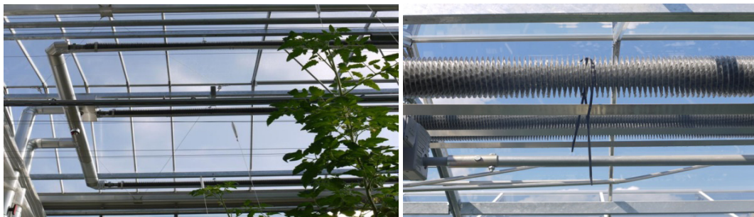
Figure 2. Heat exchangers placed under the greenhouse roof.
